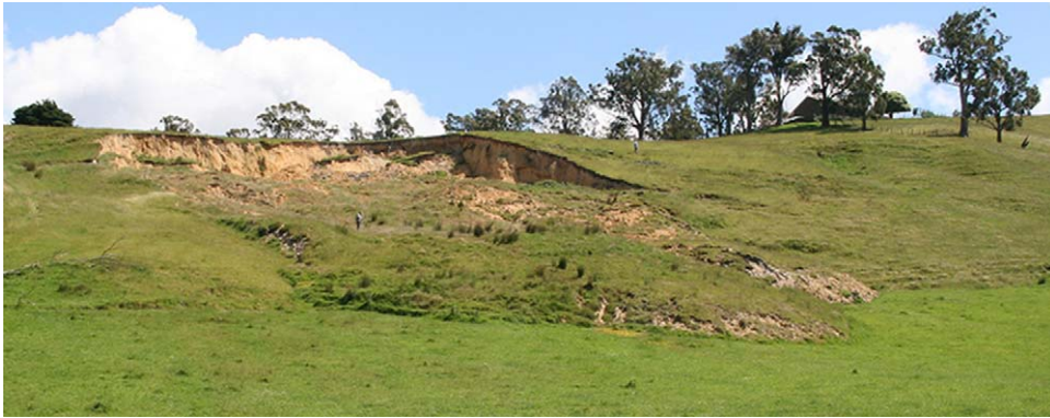
Figure 1. Overview of the Home Hill landslide located in southern Tasmania. The height of the scarp (head wall) is 4–5 m.
